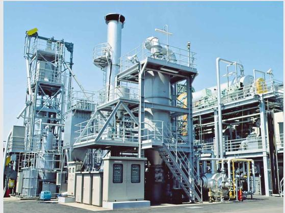
10 t/day pyrolysis gasification test facility
