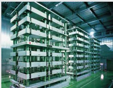
Thyristor valve for Kii Channel HVDC transmission system
